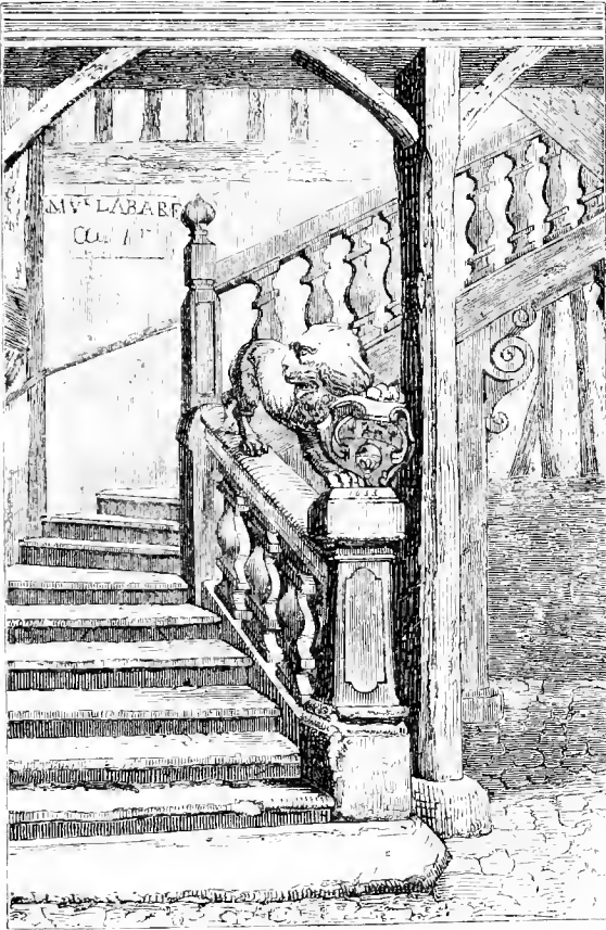
Fig. 245.—Staircase of the Office of the Goldsmiths of Rouen (Fifteenth Century). The Shield which the Lion holds with his paw shows the Arms of the Goldsmiths of Rouen (Present Condition).
